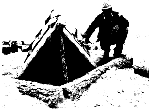
Fig. 6.4. View of the same triangular blast door, looking in a direction perpendicular to the radius from ground zero. The hinge pole, originally 7 in. in diameter after peeling, had been flattened on its top and back side. The two other poles, 8 in. in diameter, had been flattened on their bottom, top, and inner sides. All three outer poles were notched and nailed together. Note the slots between the door-covering poles.
